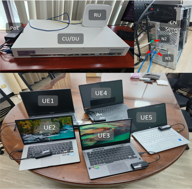
Fig. 5. (Top) The logical topology, and (Bottom) a snapshot of commercial testbed setup in L^25GC+ . RU: Radio Unit; DU: Distributed Unit; CU: Central Unit; CN: Core Network; PoE: Power over Ethernet; 5 laptops as UEs with 5G dongles
